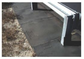
**Rubber – Not Concrete or Asphalt** Unlike concrete or asphalt aprons, Weed Mat's flexible design and construction does not inhibit the energy absorbing qualities of the guardrail post and allows guardrail post movement within the soil after an impact.
